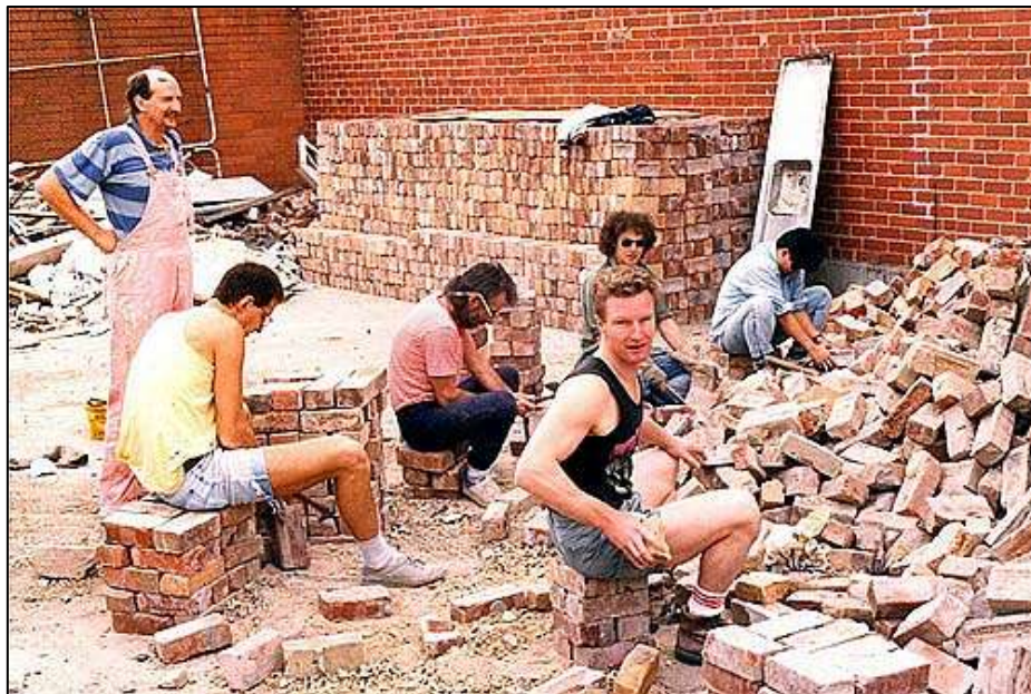
The Kenshikan under construction
