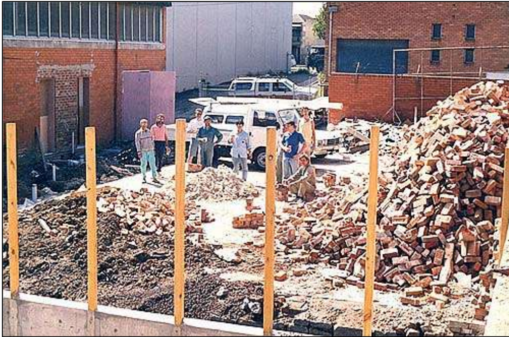
The Kenshikan under construction
